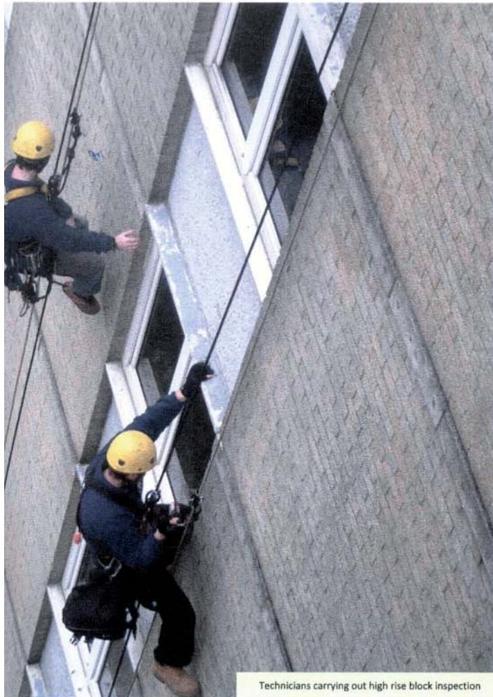
Technicians carrying out high rise block inspection
