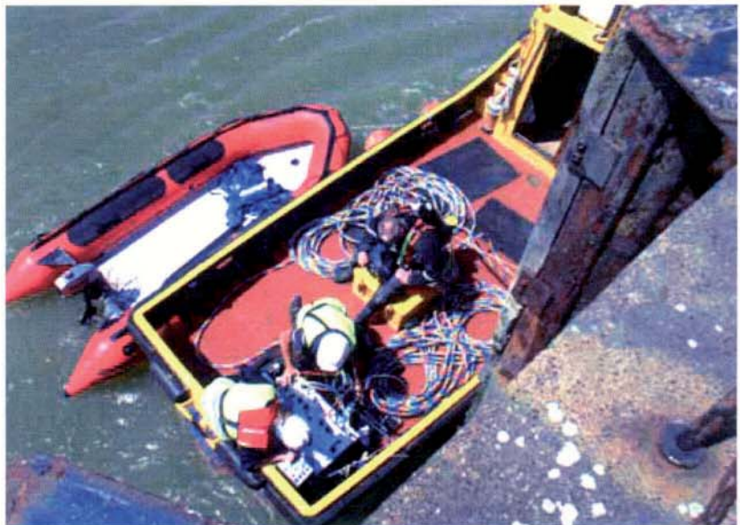
Dive team preparing for underwater structural evaluation
