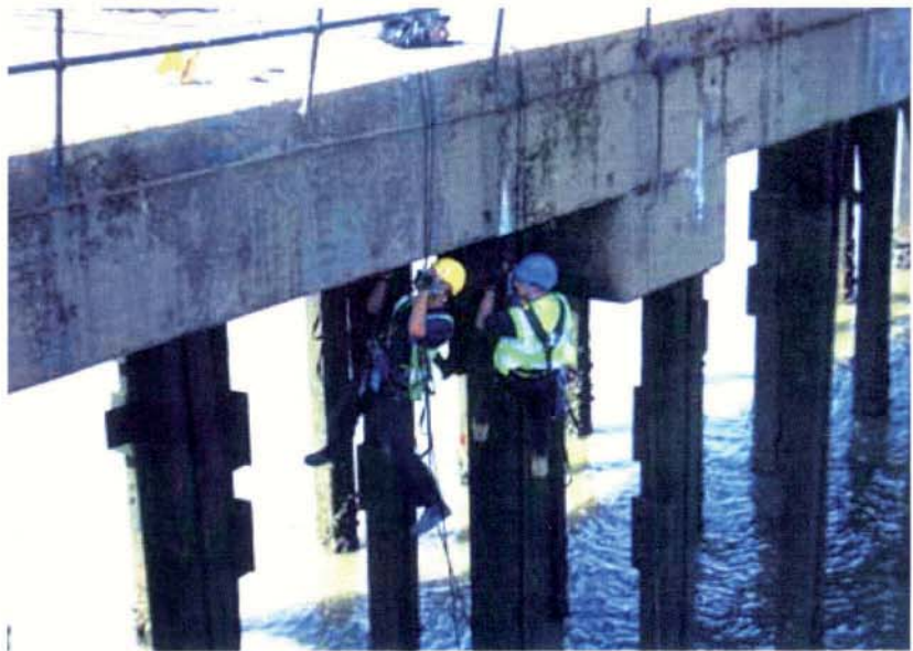
Technician carrying out survey using industrial roped access techniques
