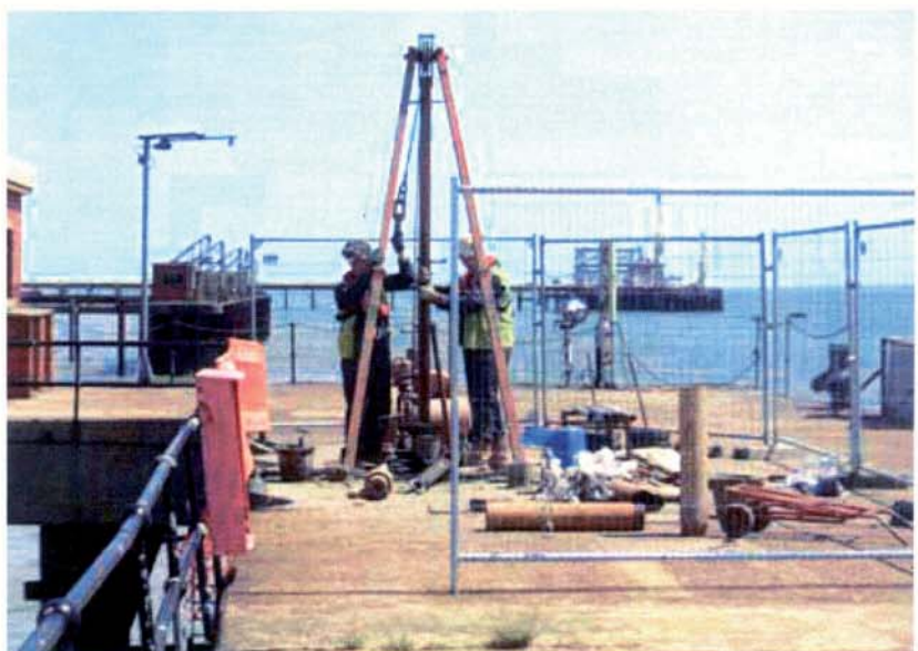
Technicians carrying out bore logging
